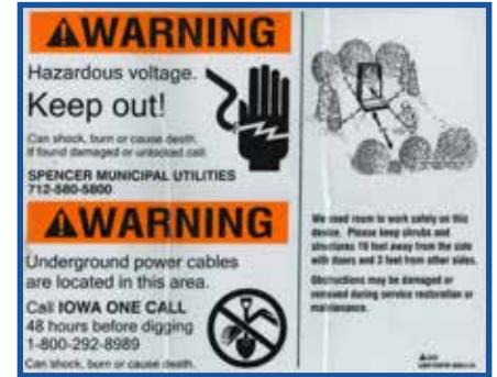
Here is an example of the warning label on the front of each transformer box. Notice they have a reminder on them regarding the space needed around them as well as the hazardous voltage warning.
